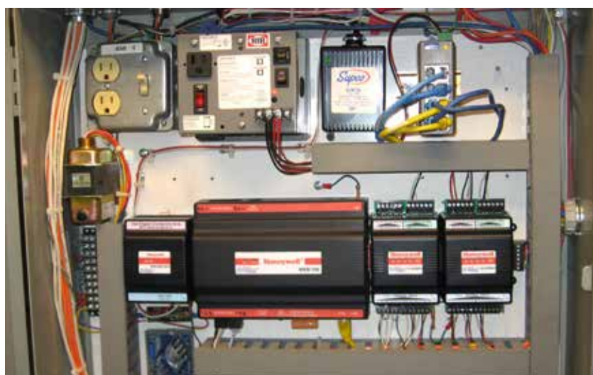
WAC's old analogue energy control system (top) was replaced by modern network-based digital controls (bottom)
