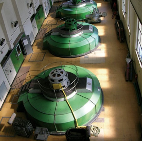
Hydro Turbines E.ON Hydro Power Station
