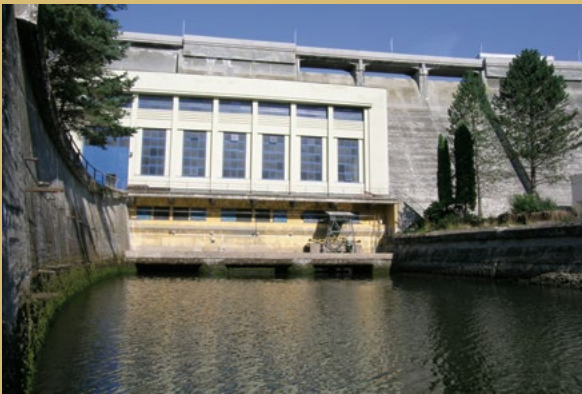
An E.ON Hydroelectric Power Plant
