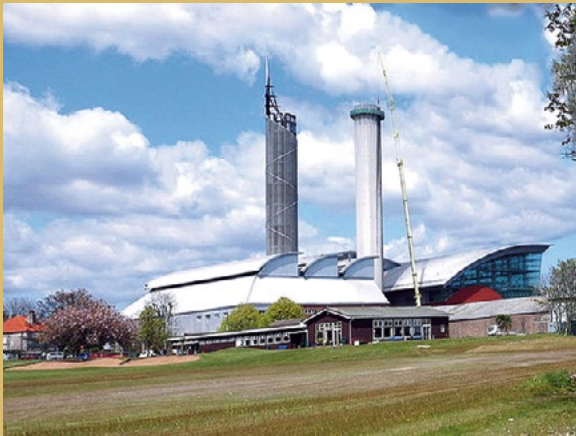
Pulrose Power Station
