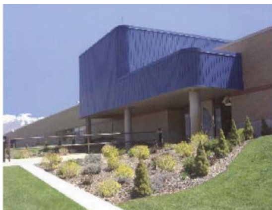
Defense Enterprise Computing Center Requires Extensive, Reliable Cooling
