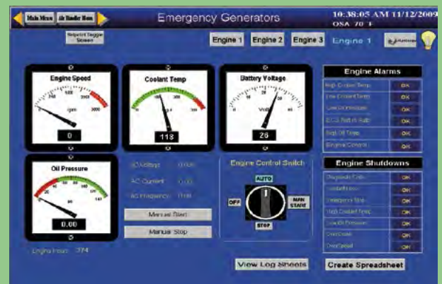
View of Emergency Generators
