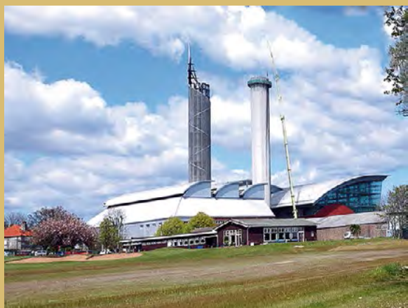
Pulrose Power Station
