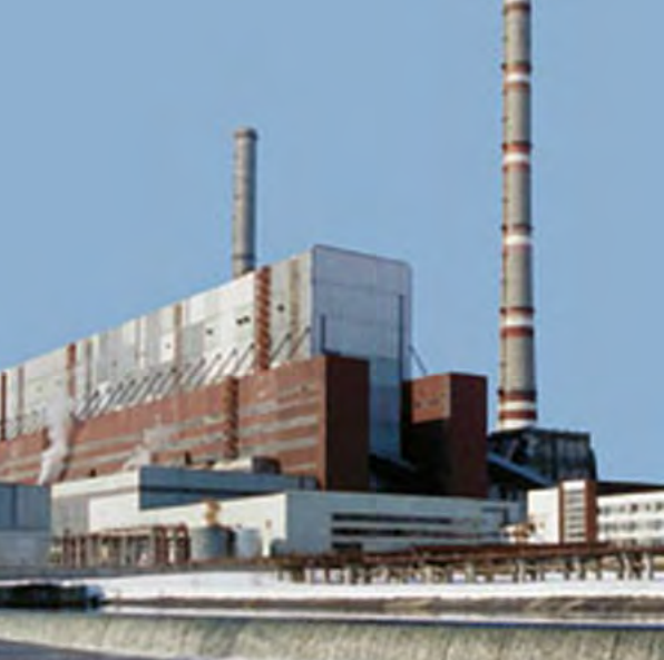
Permskaya Gres Power Plant Dobryanka, Russia
