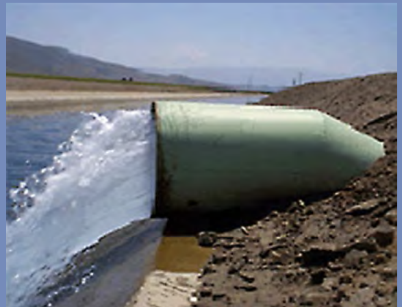
Water Transfer from Ground Storage
