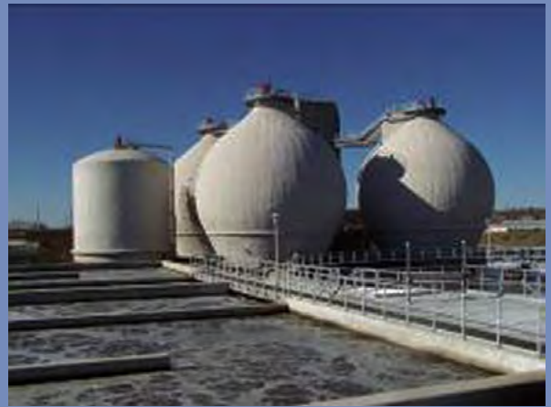
Anaerobic Digesters
