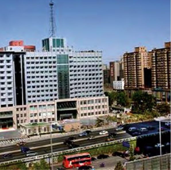
Beijing Traffic Control Center Headquarters
