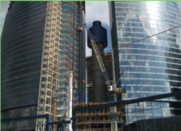
The Federation Tower Under Construction Moscow, Russia
