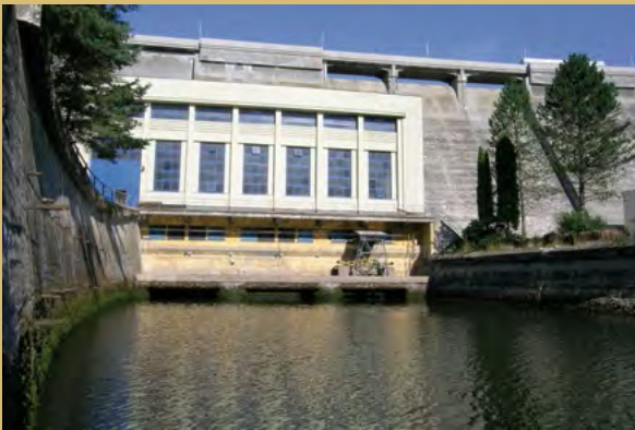
An E.ON Hydroelectric Power Plant
